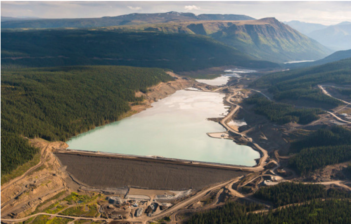
The dam at the Red Chris mine is 341 feet high. Photo Credit: Southeast Alaska Indigenous Transboundary Commission; available at: https://www.seitc.org/lakes-of-poison .
